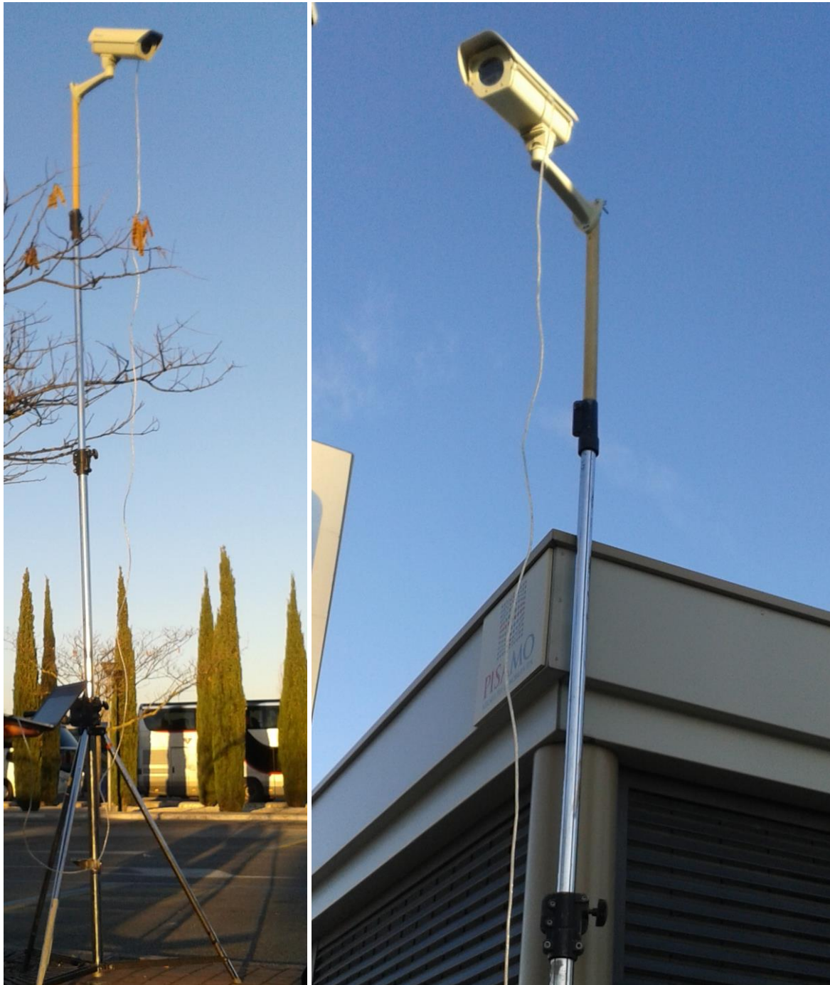
Figure 8 – Prototype installation of the parking lot monitoring devices as mounted onto a tripod.
