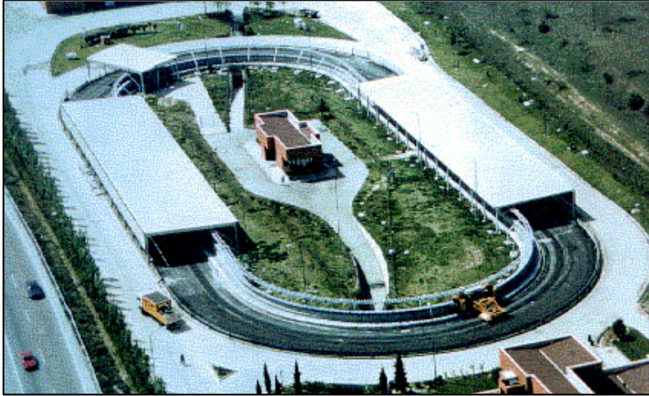
Figure 8 : CEDEX accelerated test facility (North of Madrid, Spain).
