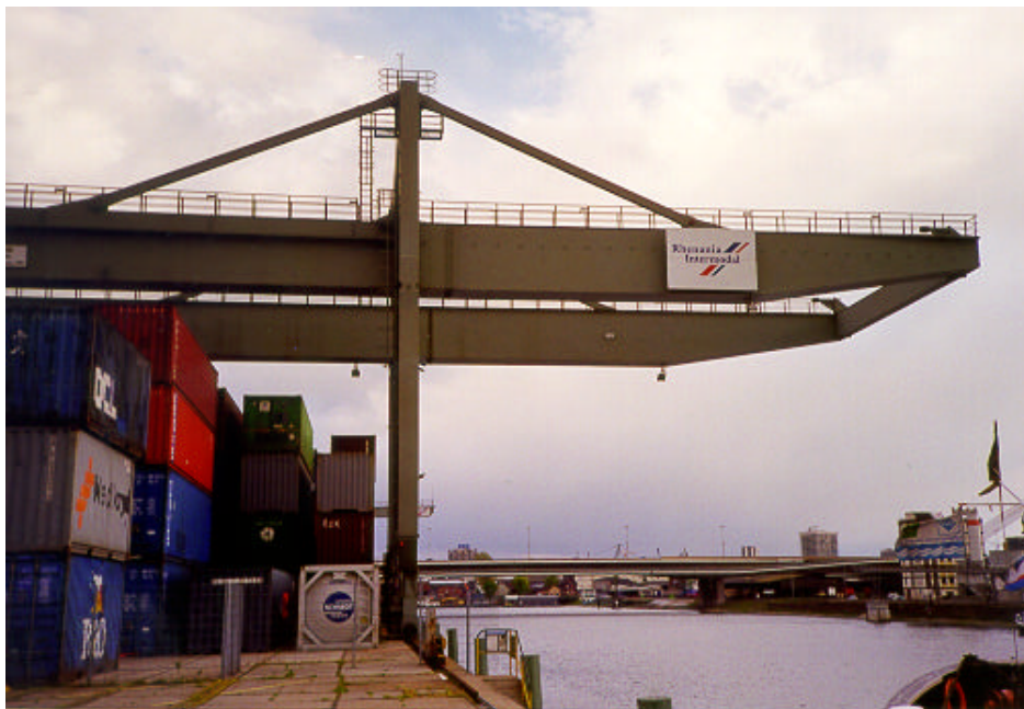
Fig. 4.3.2.1/3: Container Terminal Rhenania, Mannheim
