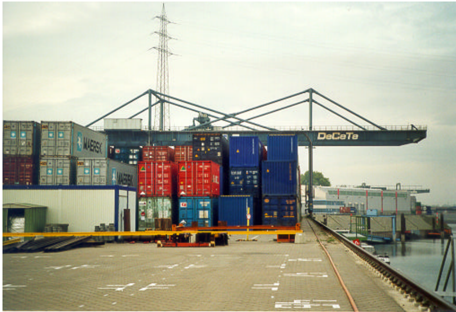
Fig. 4.3.2.1/1: Container Terminal DeCeTe, Duisburg
