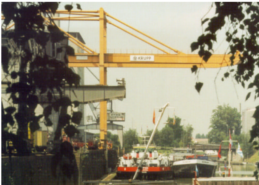
Fig. 4.3.2.1/4: Container Terminal SRN-Alpina, Basle
