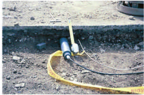
d) Installation of TDR Probe in Basecourse Layer
