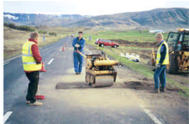
f) Compaction of Surface Dressing Layer
