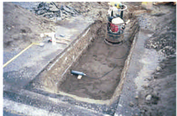
b) Sub-base TDR and Compaction Equipment
