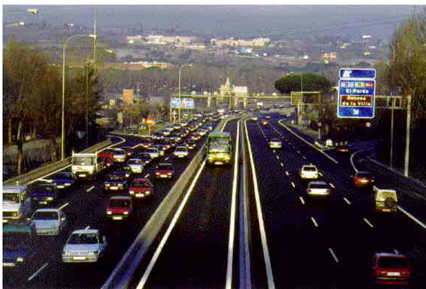
Figure 6-32: HOV lane in Madrid
