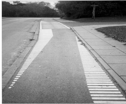
Figure 5.8. Raised crossing, Denmark.
